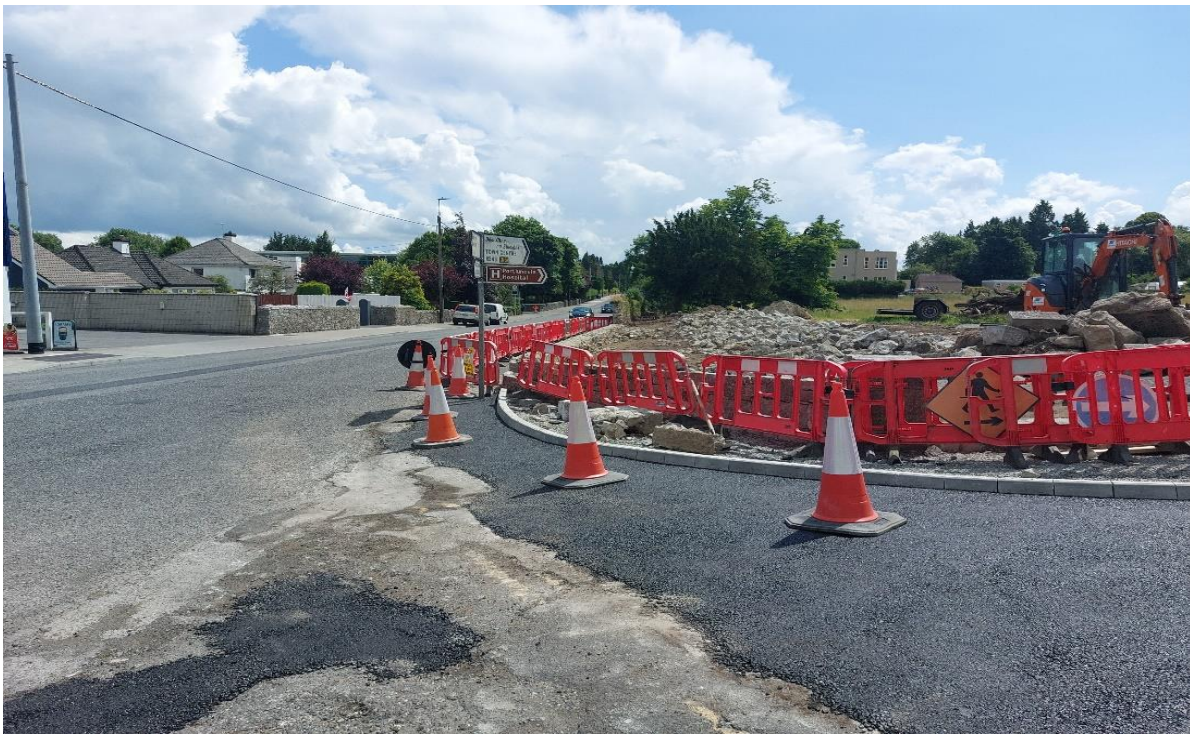
Setting back boundary walls to improve sight lines.
